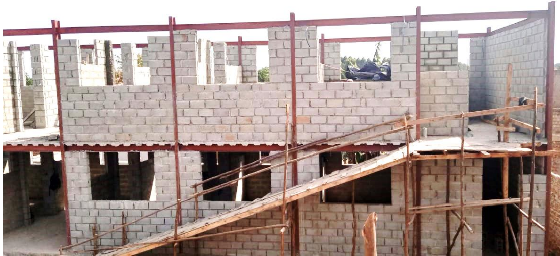
Divine Hope pupils' dormitories construction in progress
